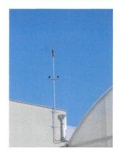
The sensors measure the outside temperature, wind direction, wind speed, solar radiation, light intensity and rain. As an option also outdoor humidity can be measured.
